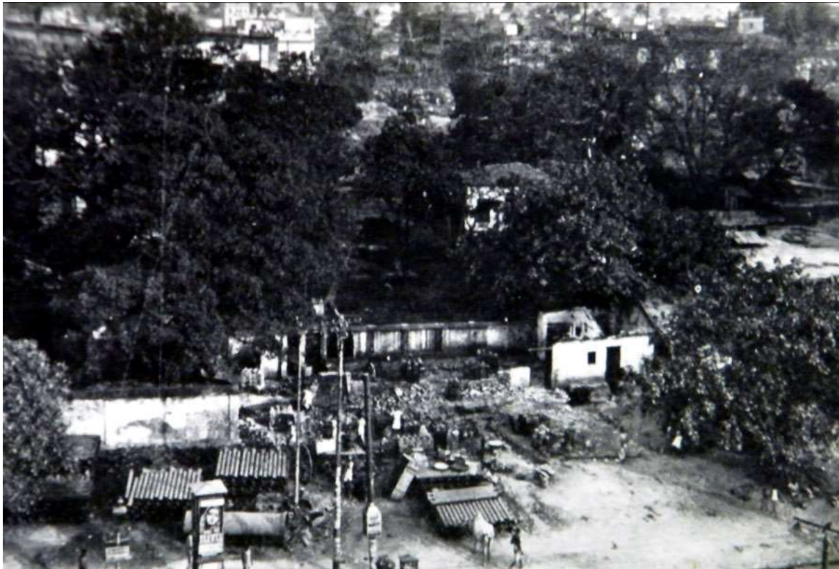
View of the scheme site, before clearance began, taken from Dharmatala Street looking eastward.
